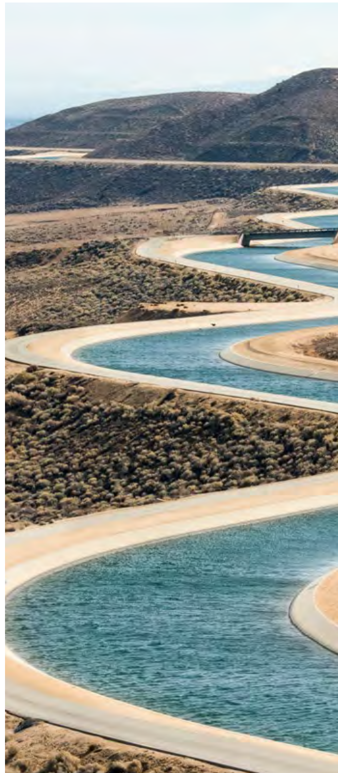
The State Water Project canal, a major conduit for imported water for the Basin.
